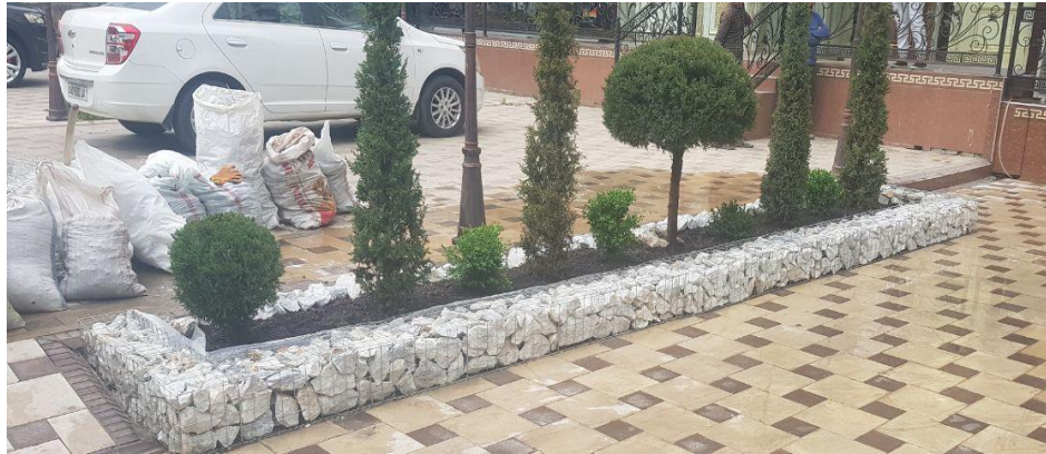
Figure 7. Building a gabion on Sebzor street
