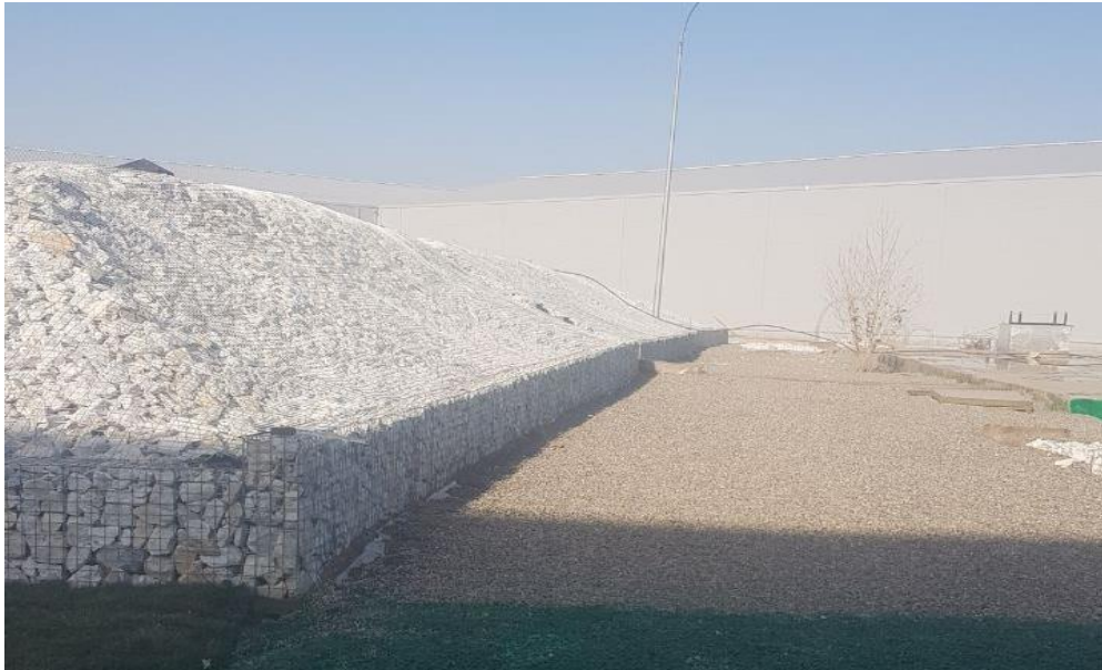
Figure 2. Use of gabions in strengthening slopes
