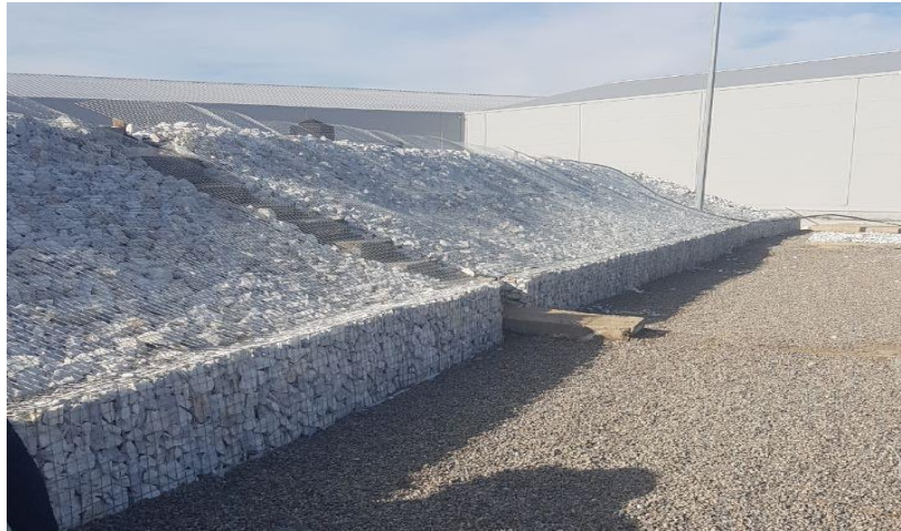
Figure 4. The finished state of gabions at "OOO BAKAN TEX".
