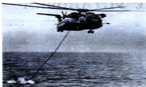
11-rasm. RH-53D vertolyotining trallash jarayoni
