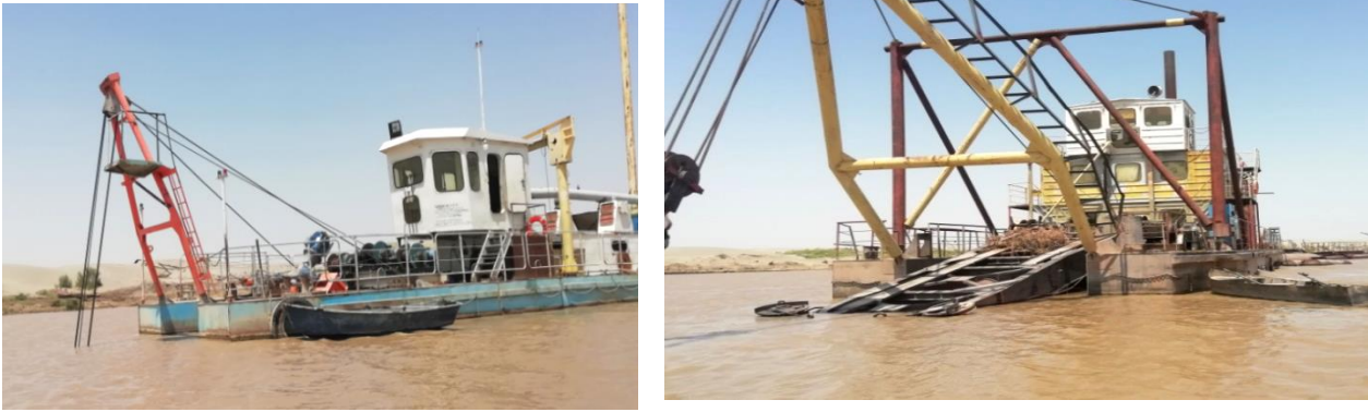
Picture 2. Zemsnaryad is in progress.
