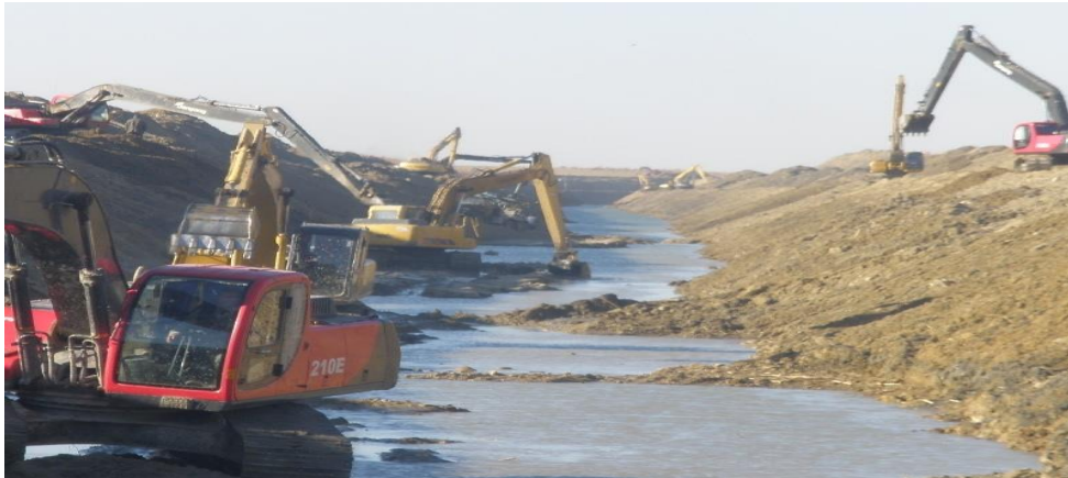
Picture 1: Excavators belonging to the State Water Special Contract Unitary Enterprise (DUK) in Bukhara undertaking drainage maintenance activities
