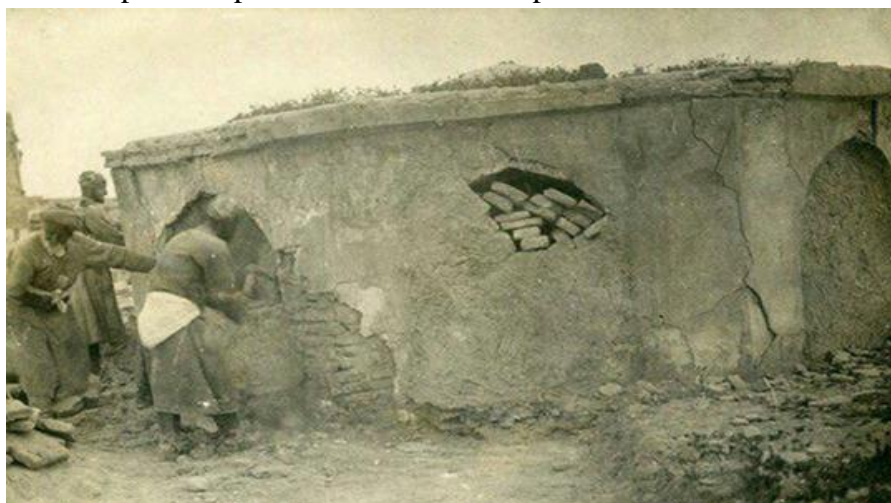
Restoration works at Magoki-Attari mosque. Dismantling repair plaster the beginning of work on. 1930s. 1934-1935
