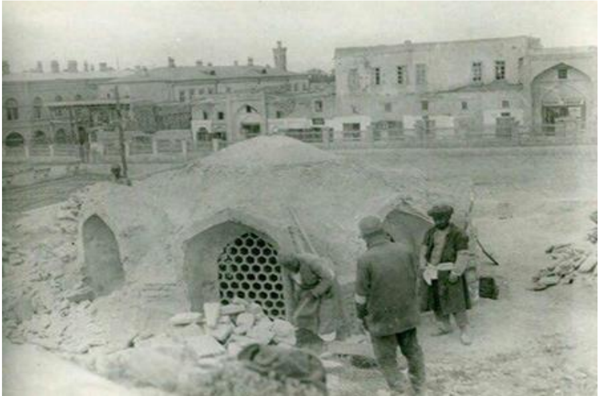
Restoration works at Magoki-Attari mosque. Dismantling repair plaster the beginning of work on making. 1930s.1934-1935
